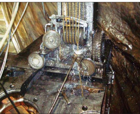
Fig 3 Hydrostress SB wire saws were supplied by Tyrolit
